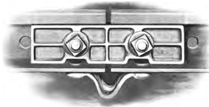
CONTACT RAIL JOINT WITH FISH PLATE
